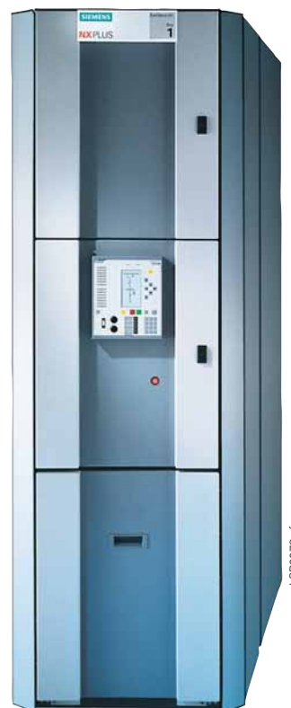
Fig. 5/122 NX PLUS panel (gas-insulated)
