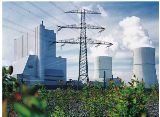
Fig. 2/13 SIPROTEC 4 in power plant application
