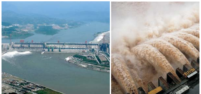
Fig. 2 Expansion stage of the dam
